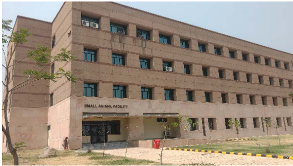
Small Animal Facility Building
