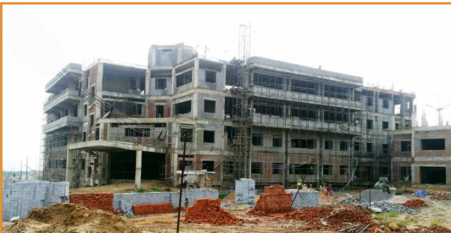
THSTI Laboratory and offices under construction at Faridabad
