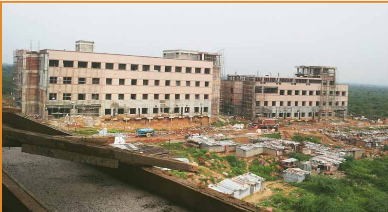
Small animal and primate research facility under construction at Faridabad
