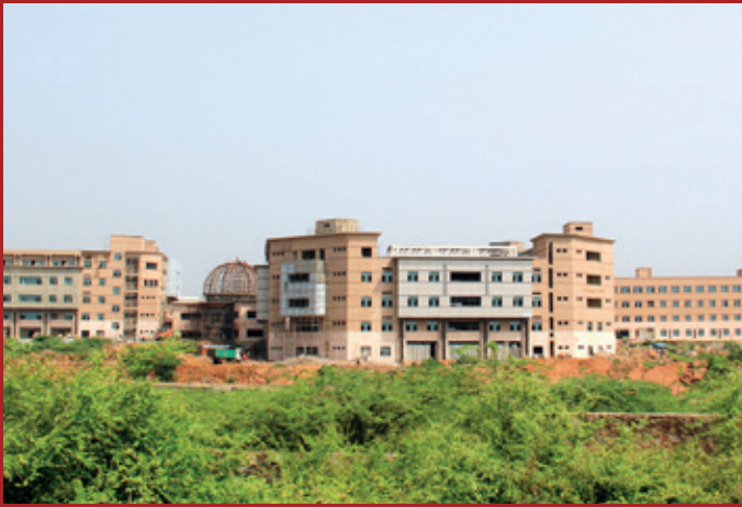
The campus under development in Faridabad
